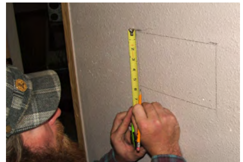
Fig. 3 Checking Hole Size
