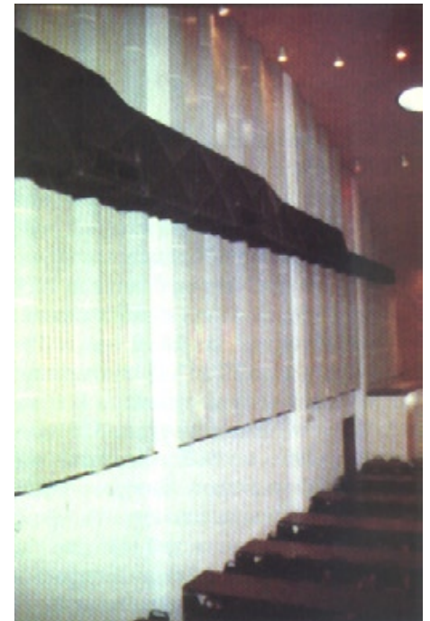
ASC TubeTraps in use at the hall.
