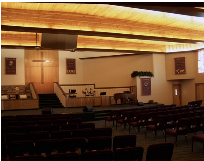
Central cluster speaker between beams
